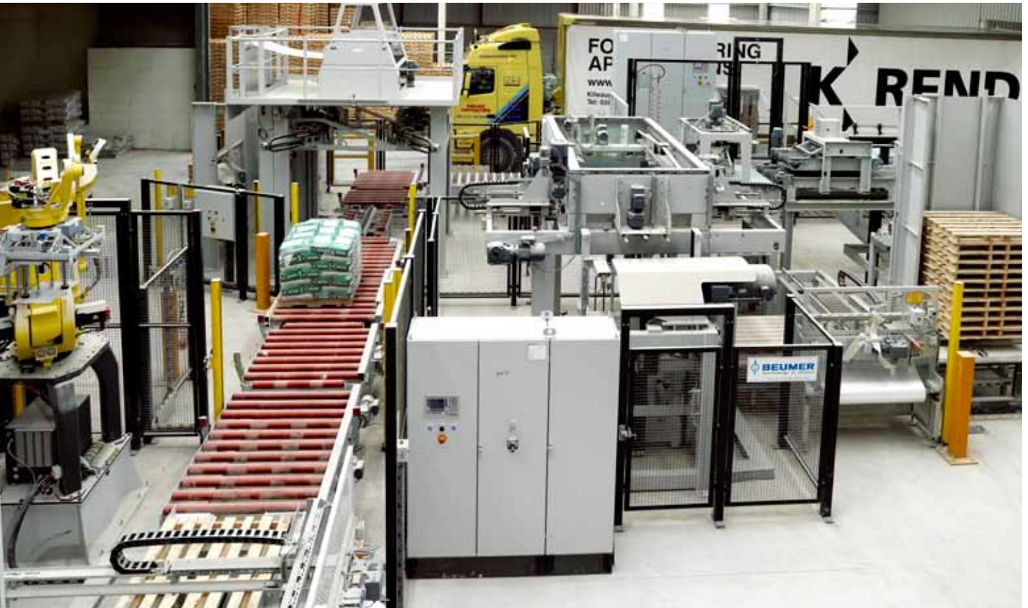
K Rend production facility
